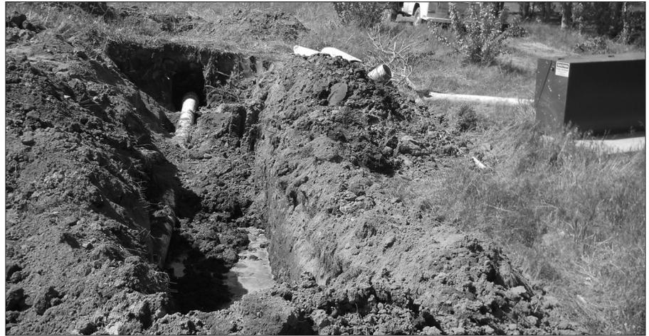
**A dig-in by a customer replacing their water line without locates. The UG transformer in the upper right had underground lines directly where the customer dug with a backhoe. Luckily, no one was injured. It was a dangerous and costly mistake for the customer.**
